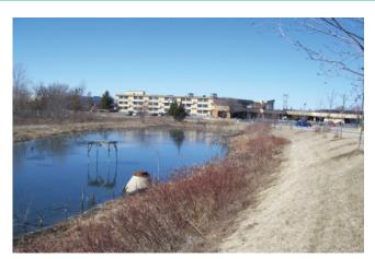
During and after wet weather, the detention pond serves as a temporary storage area for stormwater that runs off of rooftops, streets and lawns. The stormwater that enters the detention pond can become polluted with oil from cars, trash and other pollutants, which creates an unhealthy environment for humans and aquatic life. The stormwater from the pond flows to Celery Bog Nature Center where waterfowl and other wildlife can be observed by visitors.
