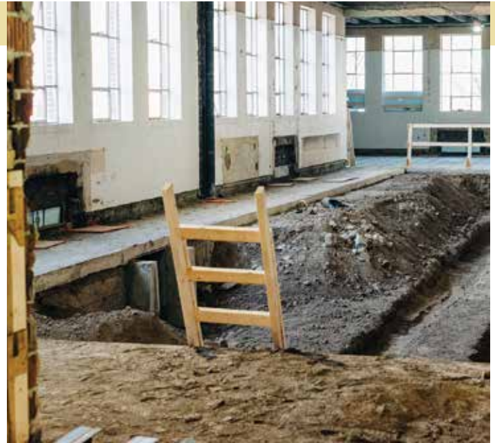
Construction is underway in the Margerum Government and Community Center.
