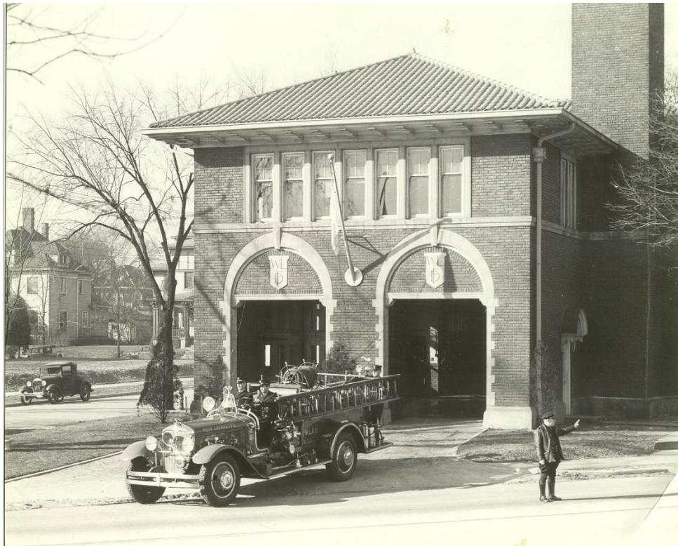
Figure 2 Station 1 est. 1917, one of Indiana's first
